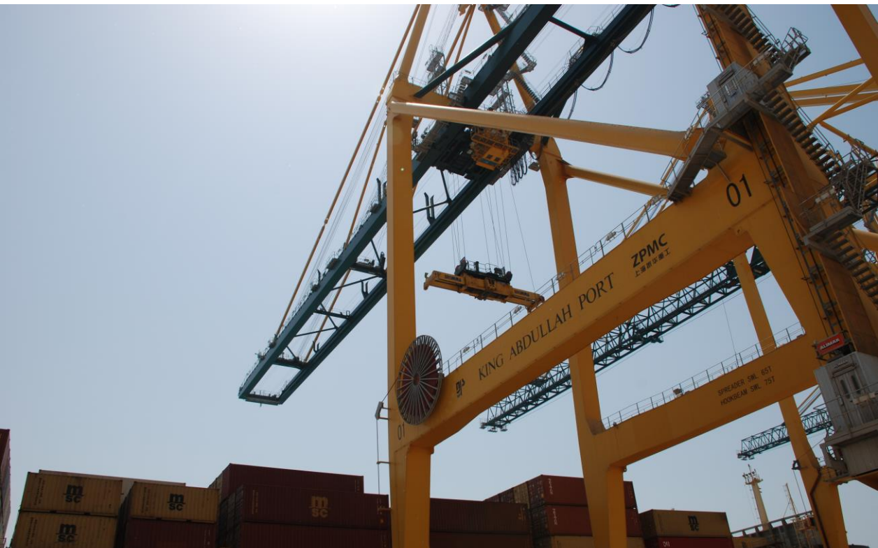
King Abdullah Port ZPMC Gantry Crane
