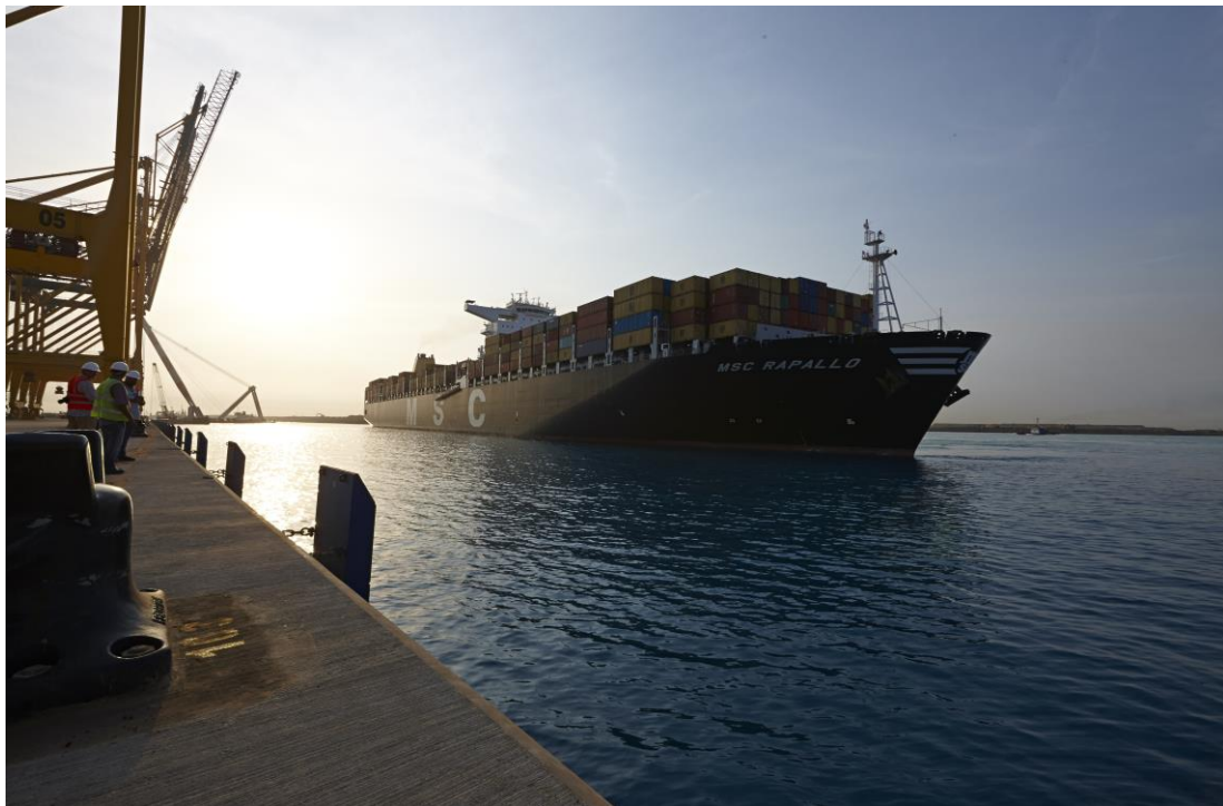
Bollard and Fender Arrangement at Berths 1 & 4
